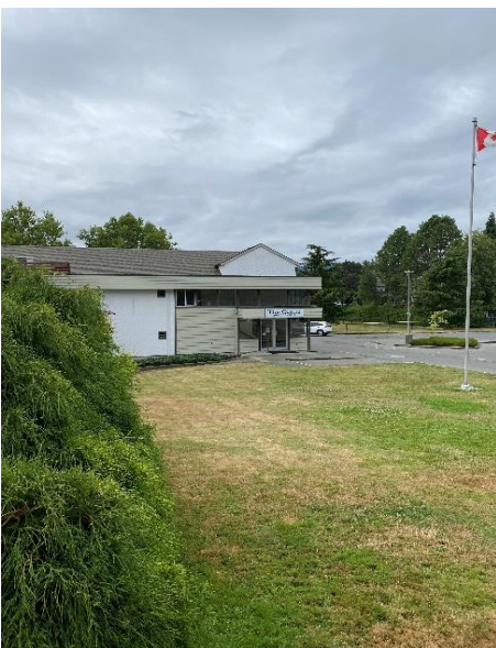
The Centre got a new paint job.
